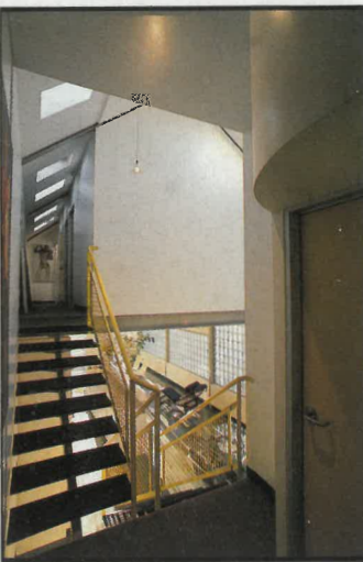
Prefabricated steel stairs, left, link the original cottage with the open-plan addition, with living areas below and private quarters above.
